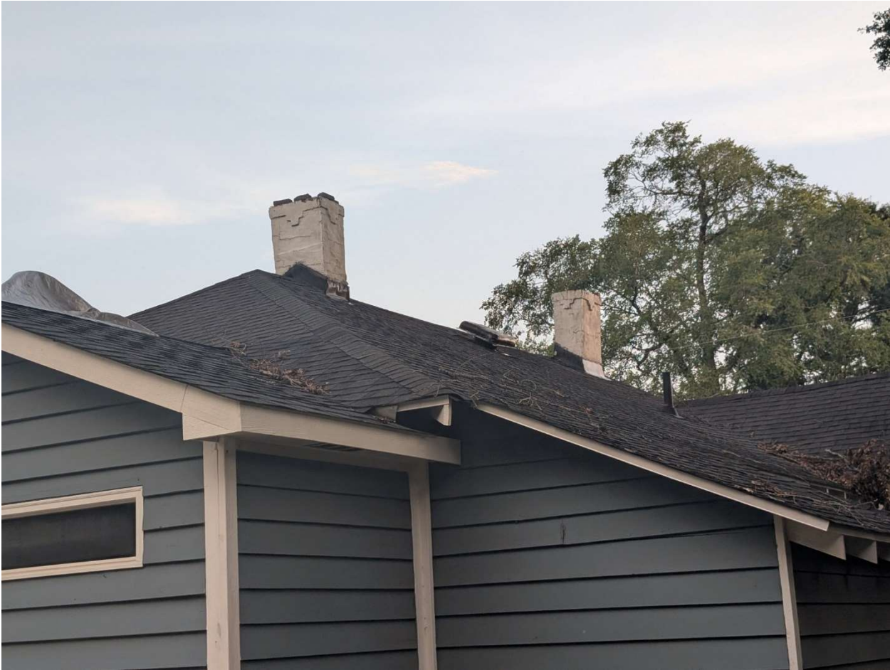
Subject property 902 Washington Street Rear Left
