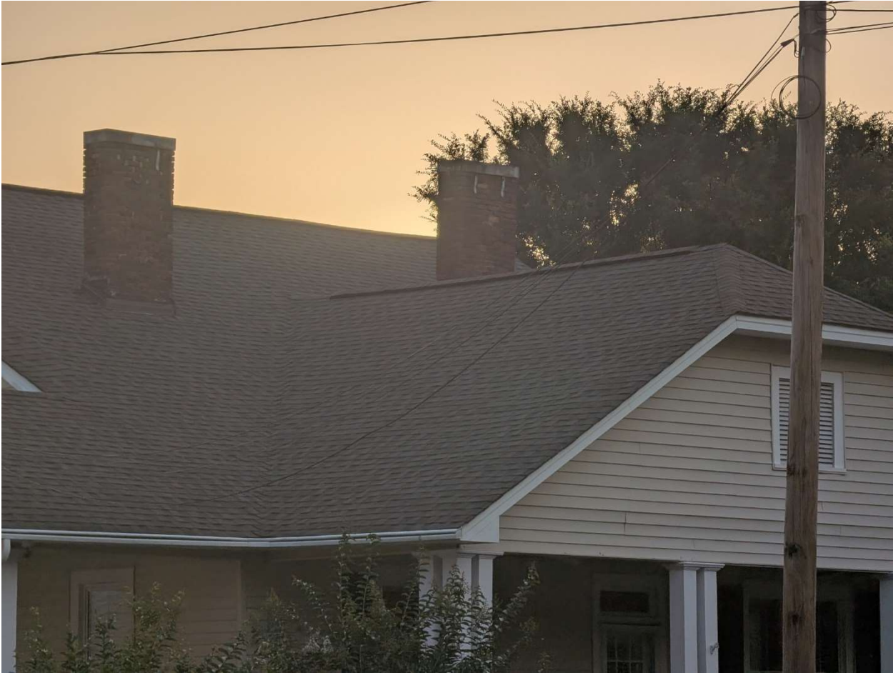
Roof of 907 Washington Street with ridge vent
