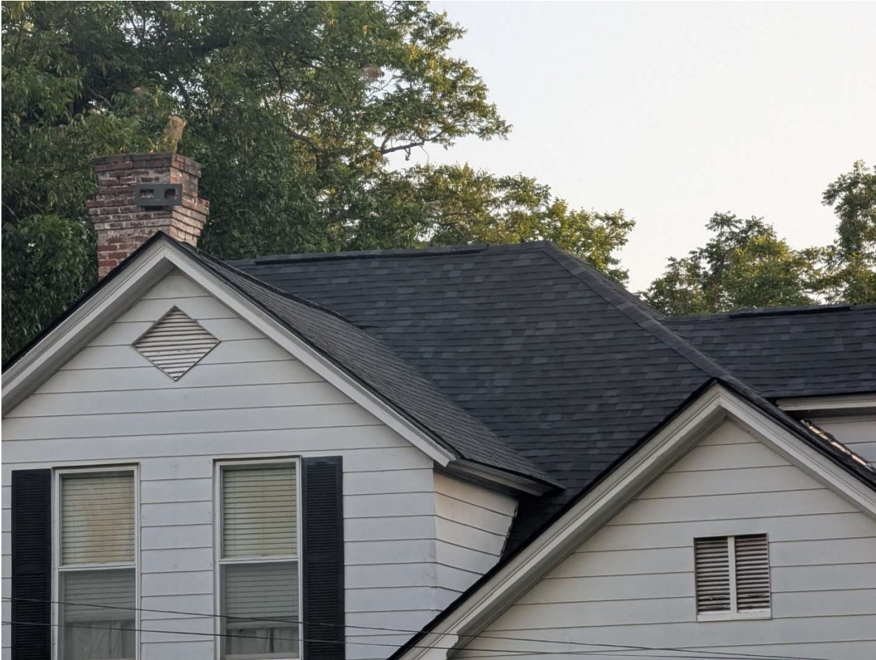
Roof of 901 Washington Street with ridge vent
